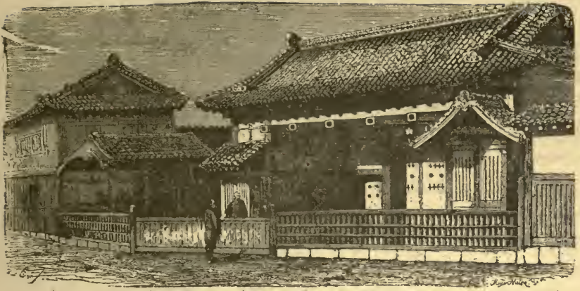
THE FRONT GATE OF THE JEWETTS' RESIDENCE.
